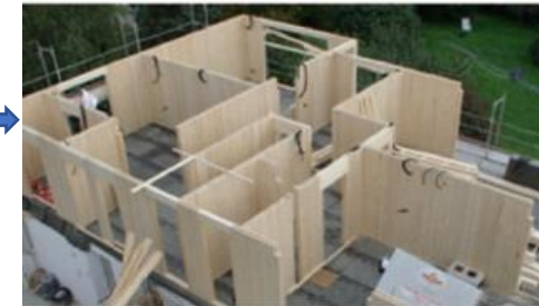
assemble room modules to whole building
